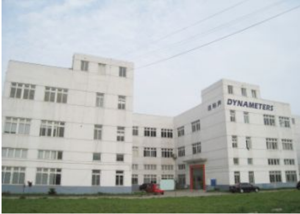
Dynaflox Office Building
